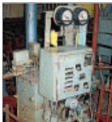
OILY VIOLATIONS: Example of an oily-water separator
