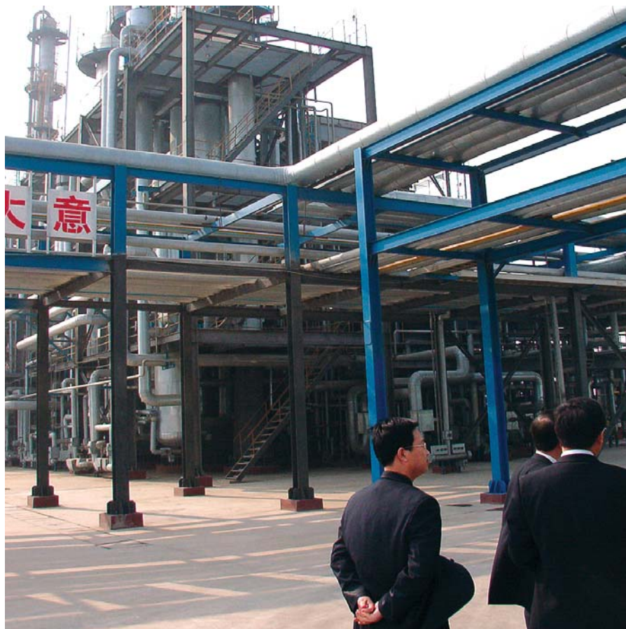
The GHU will be installed at an existing processing facility in China.
